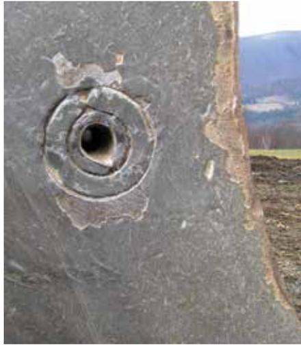
*Composite Pinning: Slotted pins are oriented 180° from each other.*
